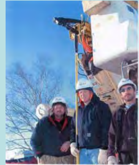
Grand Marais linemen – PCB transformer project
