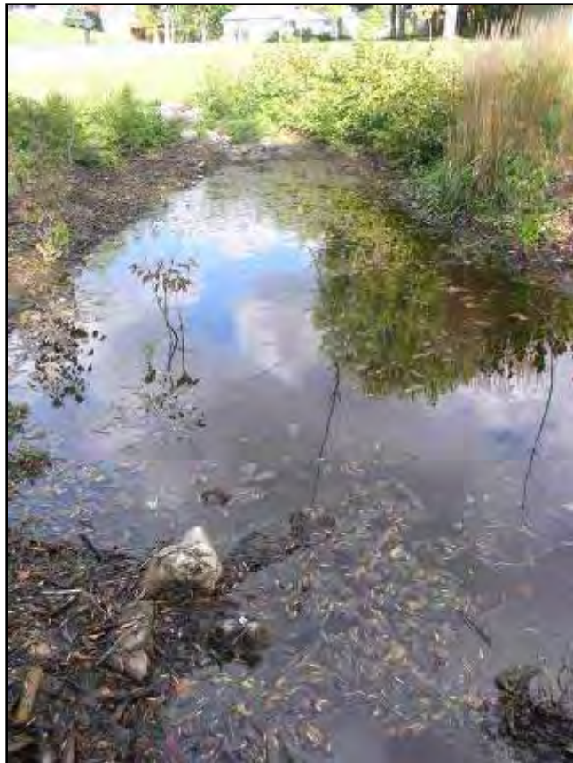
Bioretention practice (rain garden) that is not functional.
