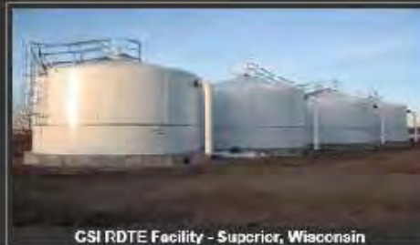
GSI RDTE Facility - Superior, Wisconsin
